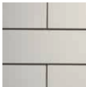
Overlapping butt joint
